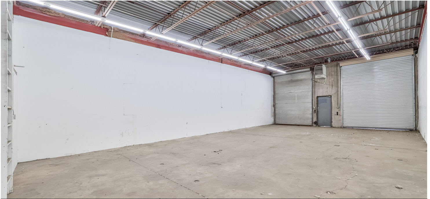
528 Rear & 529 Rear – Two overhead doors and one personnel door
