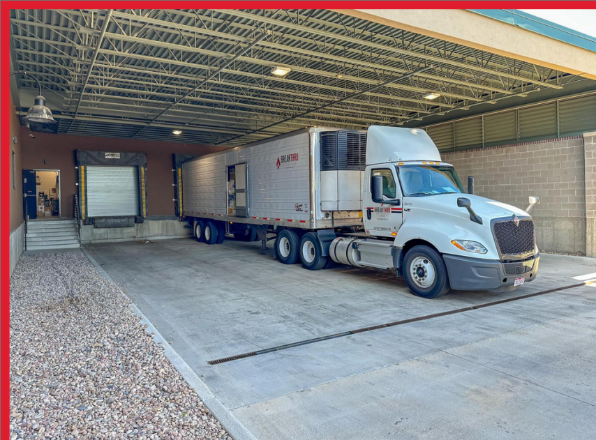
2 Covered Loading Docks - View 2
