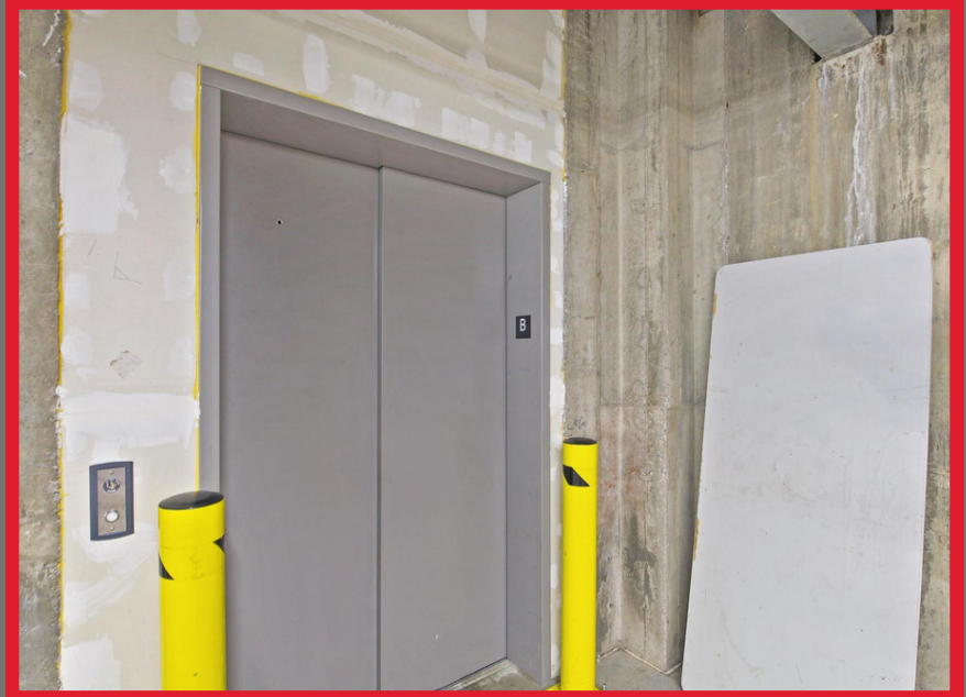
Basement Storage Elevator
