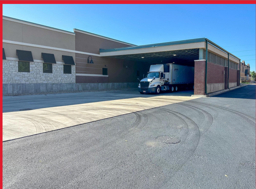
2 Covered Loading Docks - View 1
