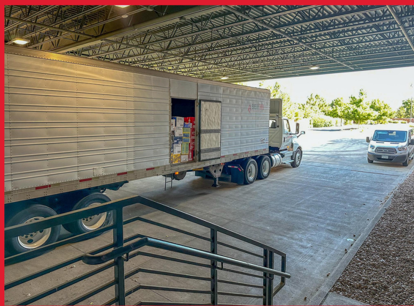
2 Covered Loading Docks - View 3
