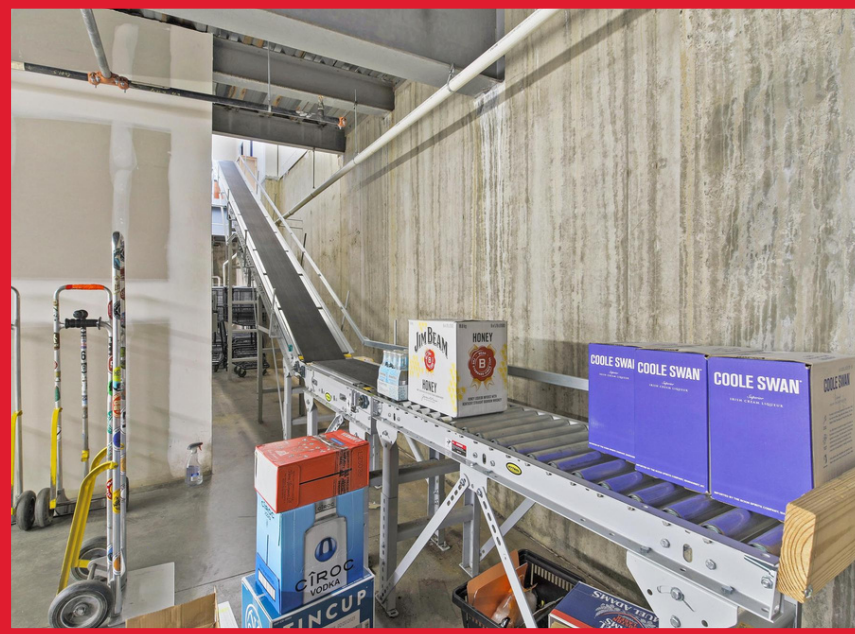
Basement Storage Conveyor Belt
