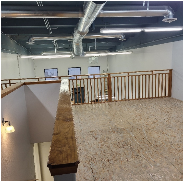
Mezzanine/storage & utility equipment
