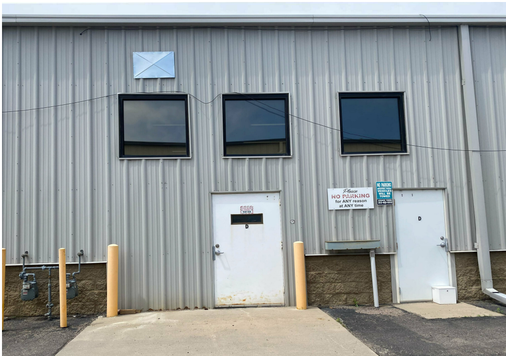
Two doors to unit production space
