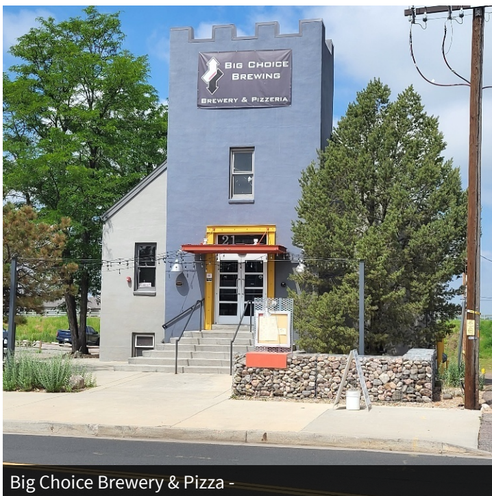
View of building from park
