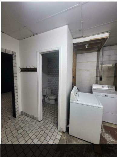
Restroom and Laundry
