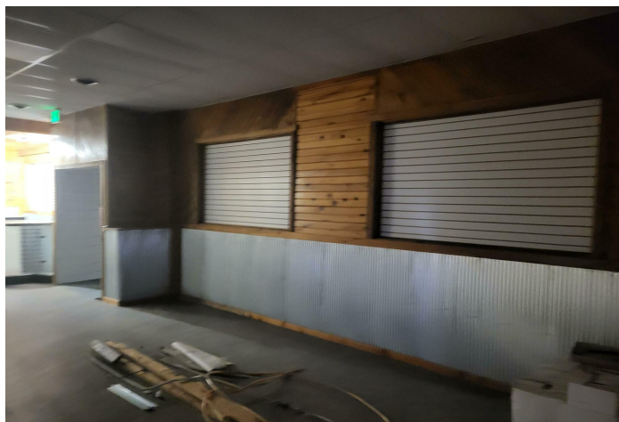
Main Room Secured Windows
