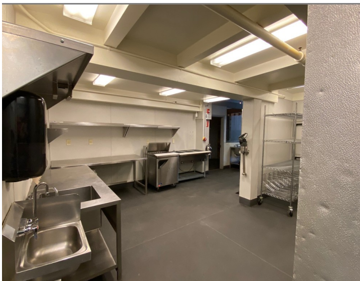
Chopstickers Unit 101 Back Kitchen
